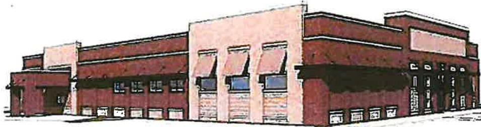
Figure 6-6-3: Awnings along a public sidewalk
