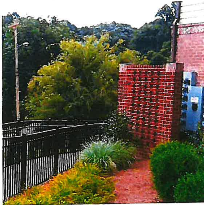
Figure 6-7-5 Service area screening
