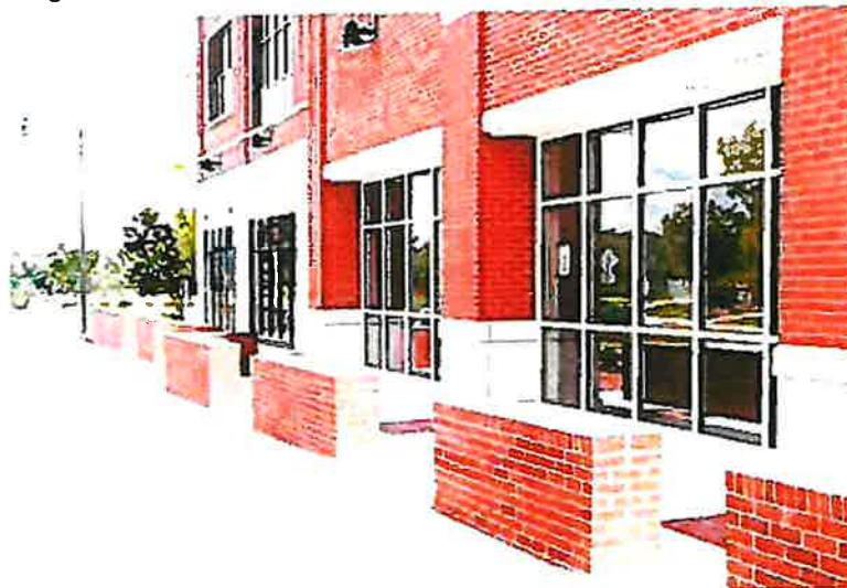
Figure 6-6-6: Facade transparency (windows) along a street facade
